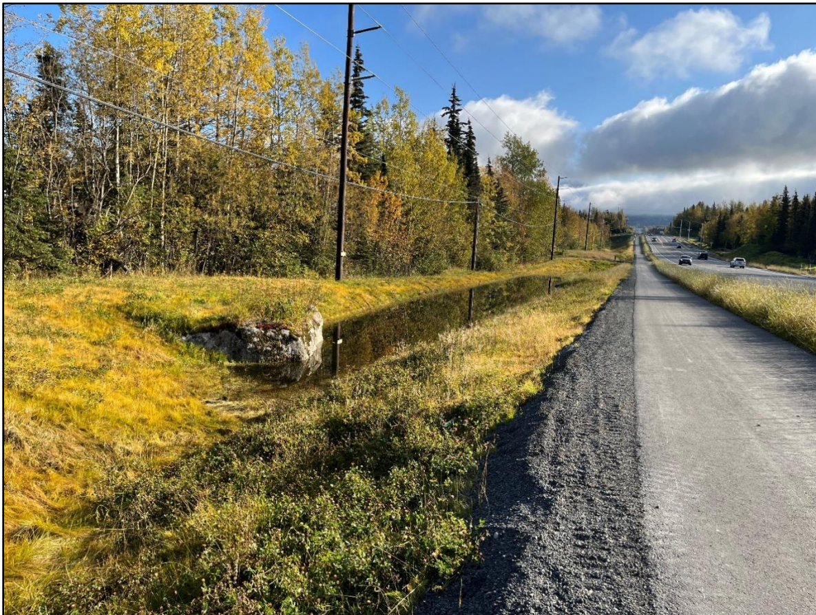
O'Malley Infiltration Basin, looking east toward Elmore Road
