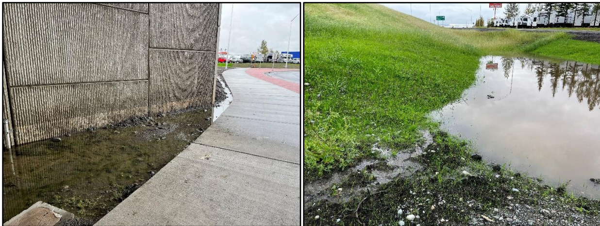
Figure 4: Groundwater Inflow to Pond D03
